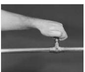
24. Open main water supply shut-off valve. CHECK FOR LEAKS! Close previously opened faucet (step 15).
