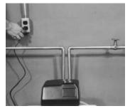
23. Plug cord from control valve into a 115V grounded electrical outlet. Make certain that outlet is supplied with power at all times. Make sure area is dry before plugging the unit in.
