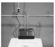
18. Typical finished installation using rigid copper pipe. Make sure bypass is in the service position to ensure household service of treated water.
