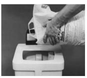
29. Pour salt into compartment. Fill about 3/4 full initially. Do not pack full. This is also where iron control salts will be put if you have rust stains.
