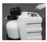
28. Measure 1-1/2 oz of chlorine bleach and pour solution directly into the brine tank. (Required on initial installations only.) Manually regenerate the softener by pressing the extra cycle button for 8 seconds to run bleach through the softener.
