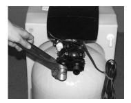
13. Check inlet and outlet for correct water flow by matching arrows on valve head and on manifold (especially if replacing existing unit).
