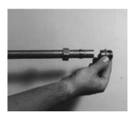
17. Soldering is no longer required to plumb with copper pipe. Instead use compression fittings. Connect plumbing as required for the specific application.
