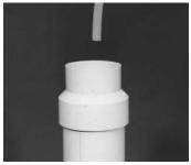
21. Typical drain line ran into stand pipe with proper 4" air gap. NOTE: An air gap is required by most local plumbing codes to prevent waste water back flow. Check and follow your local codes.
