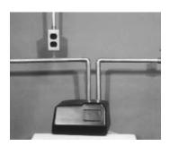
9. Position softener near the main water supply line, a drain, and an electrical outlet. Position so that main water supply shut off valve is between the softener and the main water source. NOTE: Install unit in an area protected from the elements and freezing.
