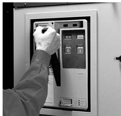
Through-the-Door Design for Human Interface with the Breaker Compartment Door Closed, for Example, Manually Charging the Stored Energy Springs
