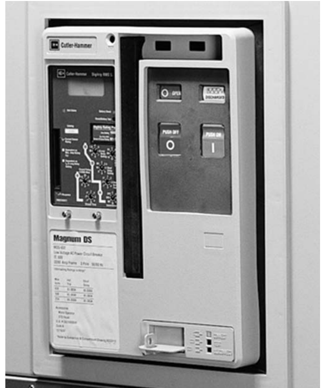
Through-the-Door Design for Human Interface with the Breaker Compartment Door Closed
