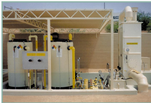
Material of Construction: UV Stabilized Polyethylene Application: Pump Station Problem: H 2 S Solution: 1,000 CFM Low Profile PT512-MD Packaged System
