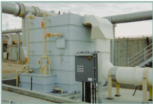
Material of Construction: UV Stabilized Polyethylene Application: Headworks Problem: H 2 S Solution: 12,000 CFM Low Profile PT512-MD Packaged System
