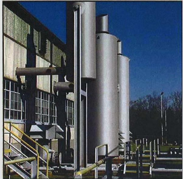
High temperature compressor mufflers operating at temperatures up to 900°F (482°C), coated with the TSA Corrosion Protection System.
