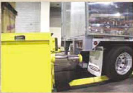
Height alignment system adjusts trailer into its proper position.
