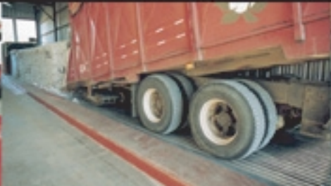
Curb poured around a floor system.
