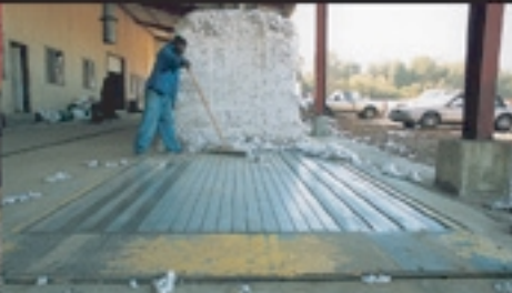
Flush mount with concrete.
