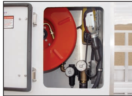
Close-up view of the hose-reel/FLR compartment.
