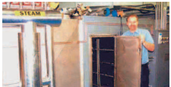
The steam system was kept in place for back-up
