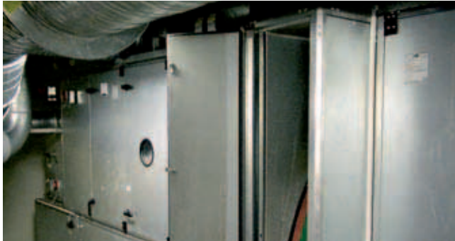
Air handling unit with heat recovery wheel, return air in the top, supply air in the bottom.
