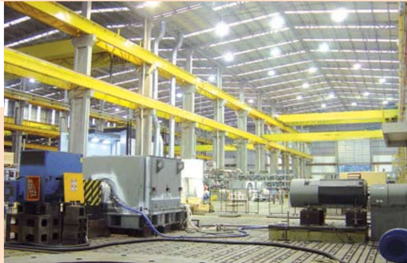
20 MVA Test Lab
