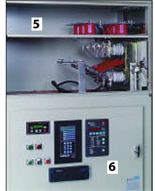
**7.** Specified surge capacitors and lightning arrestors. TECO–Westinghouse Motor Company can design, mount, and test (as an integrated unit) surge capacitors and lightning arrestors to match your electrical system and lightning protection requirements.
