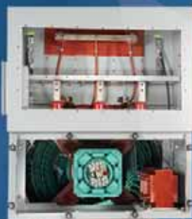
High Voltage with Rear Cover Removed
