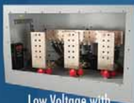
Low Voltage with Rear Cover Removed
