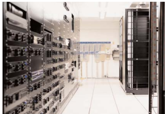
Emerson Network Power's approach to servicing your critical space covers all aspects of availability and performance, from individual power and cooling equipment to the entire mission-critical system.
