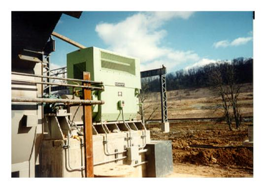
The LSC design also includes a three way valve for filter bypass or filter changeover, flanged connections for oil supply and return, three way back pressure regulator to adjust oil flow rate (factory preset) to motor bearings and large clean out doors on each end of the reservoir. Included as standard are connections for oil purifier and nitrogen or oil mist purge.
