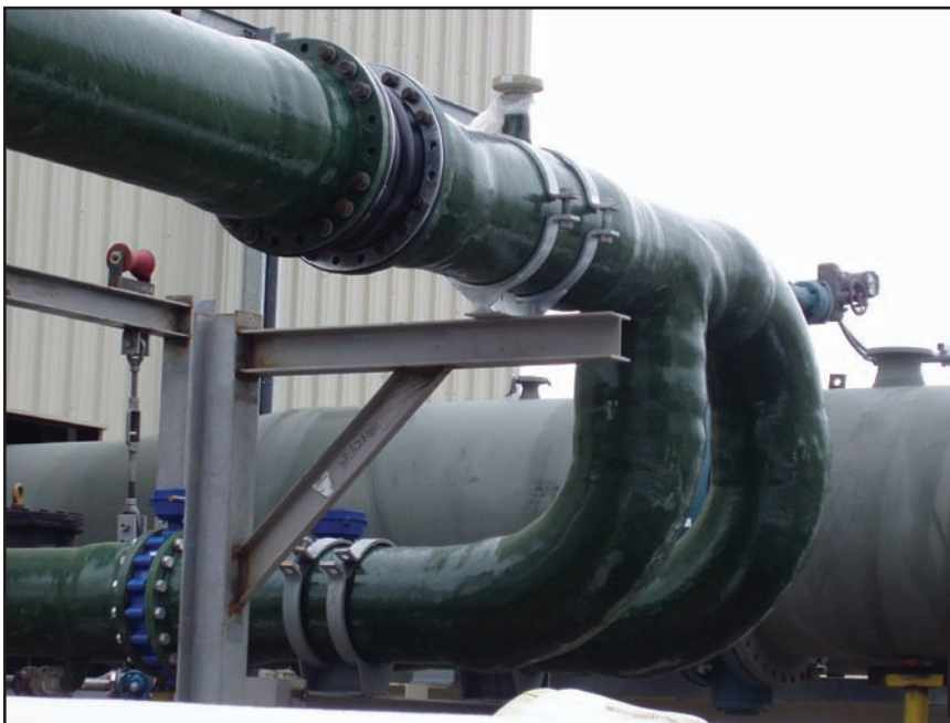
18-20 inch diameter recirculation water application in Salt Lake City power plant
