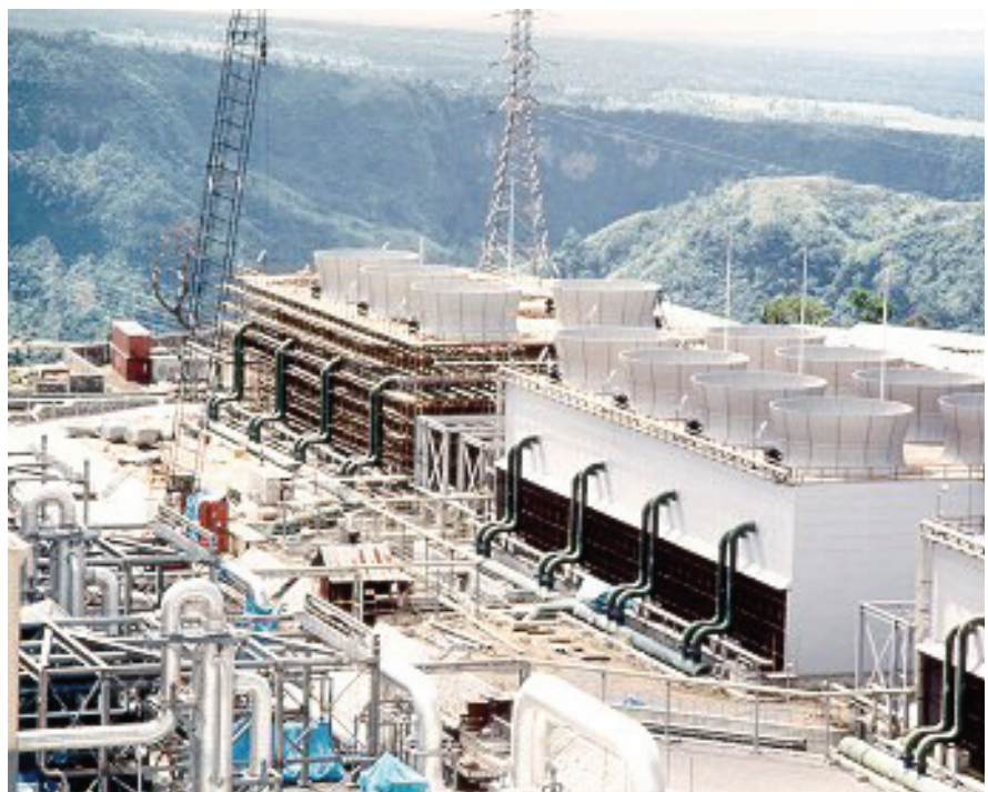
16-72 inch diameter cooling water piping installed at Fuji Electric, Philippines
