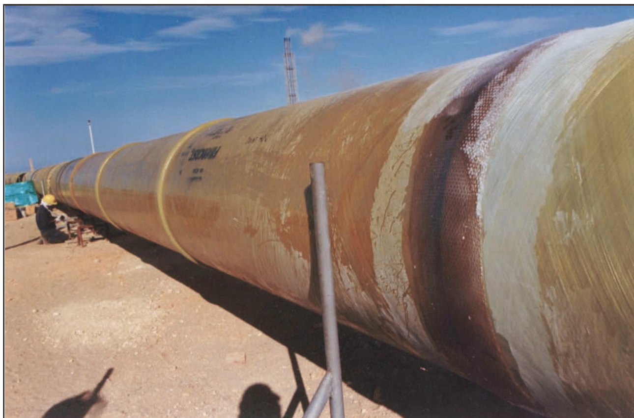
VENEZUELA: 60-INCH EPOXY RESIN PIPE FOR PROCESS WASTE AT A REFINERY
