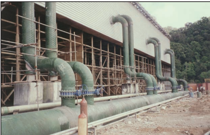
Power plant condenser water return lines
