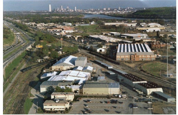
Sand Springs, Oklahoma Facility 172,000 sq. ft. manufacturing space
