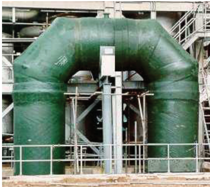
60-inch cooling water recirculation lines
