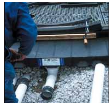
All Center and Side Track Pans are molded with pipe fitting locators at their lowest point. Below-grade piping can be installed to channel large spills to oil/water separators, holding ponds, etc.
