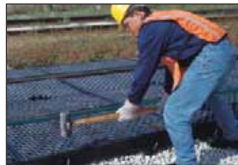
Side Pans are secured in place with rebar or other fasteners. (2-foot-long rebar fasteners with protective caps are available as options.)
