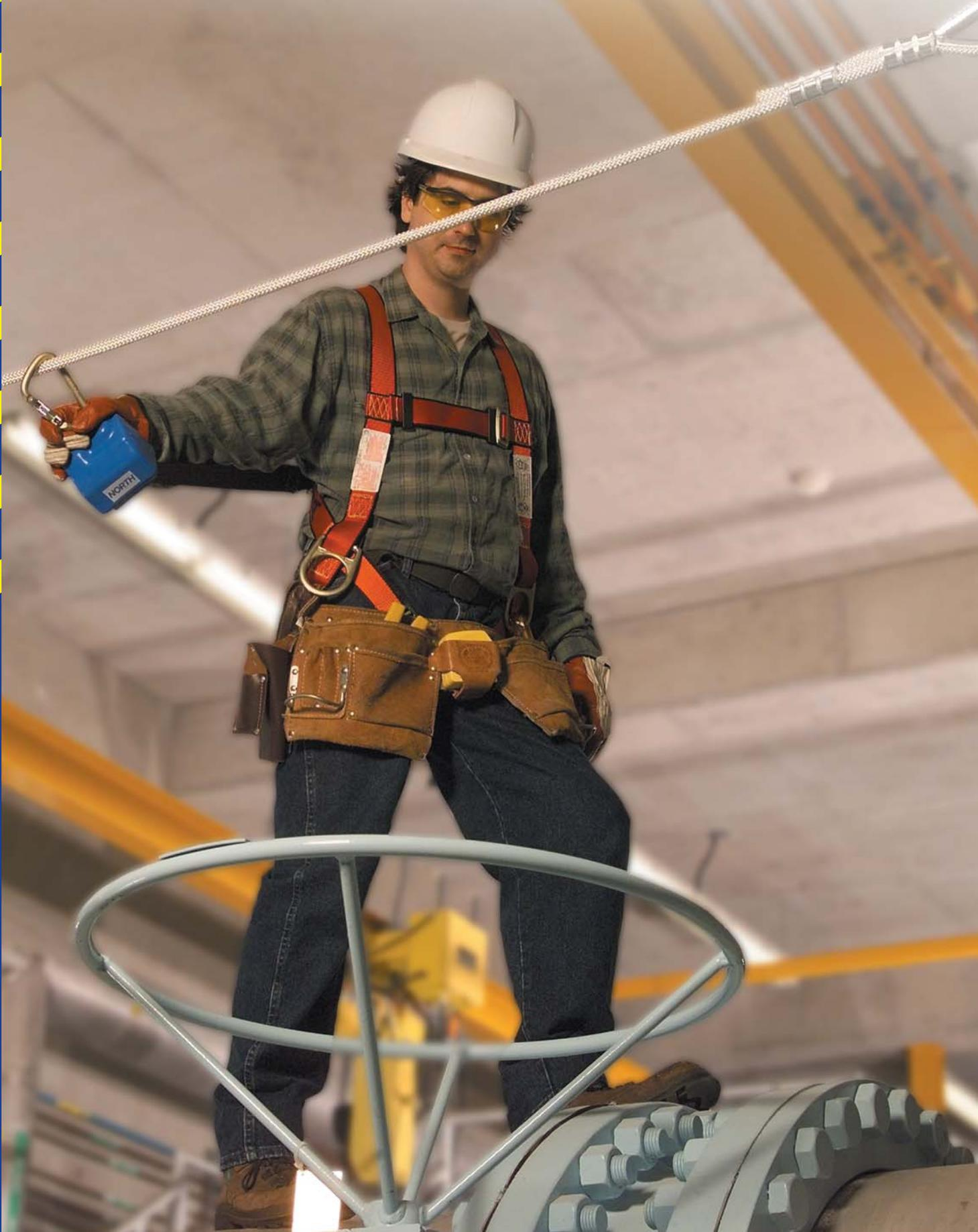
Safety and mobility – these are the hallmarks of North’s Temporary Horizontal Lifeline (HLL) Systems. Whether rope or cable, these systems provide durable protection that can be moved from site to site where there are suitable approved anchor points. 100% portable and lightweight, these systems are ideal for the construction job site or bridge and building inspection activities.
