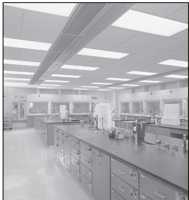
Short-Throw Diffusers with Exhaust Hoods
