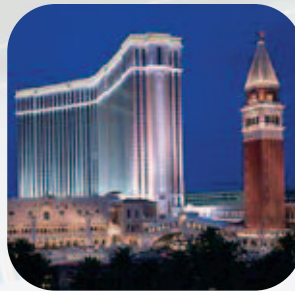
Bell & Gossett 70M, four pump constant speed pressure booster, in The Venetian Las Vegas, Nevada
