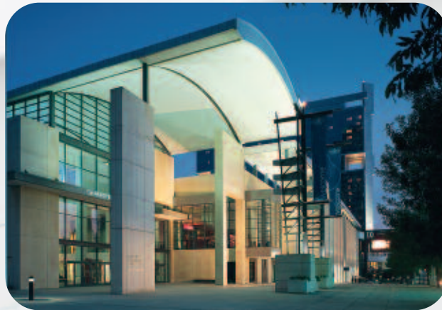
Bell & Gossett Powersav System controlling 22 zones in Charlotte Convention Center in Charlotte, North Carolina
