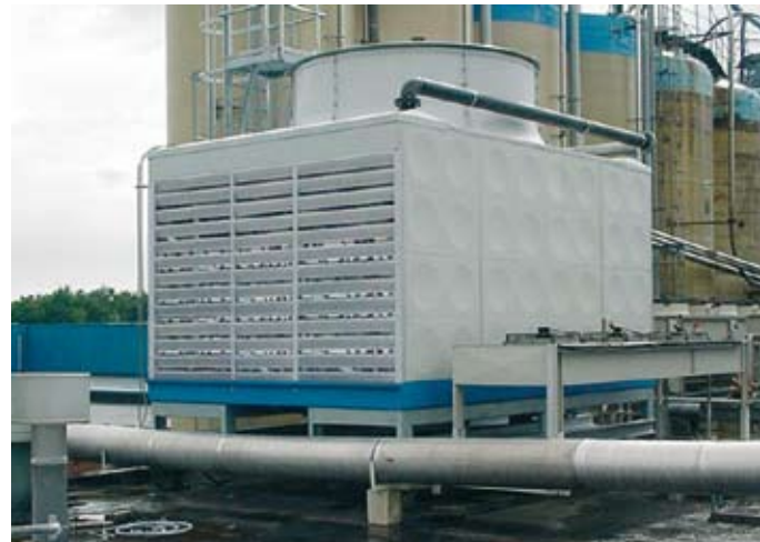
Cooling Tower type XL 2.320 Chemical Plant in The Netherlands
