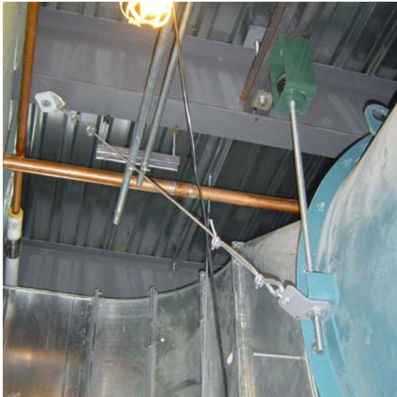
For large suspended equipment, spring hanger vibration isolators (Vibro-Acoustics Type SH) are used on each support rod to absorb the equipment vibrations. To deal with the anticipated seismic forces, both lateral and vertical bracing must be installed in such a manner as not to hinder the effectiveness of the isolators.
