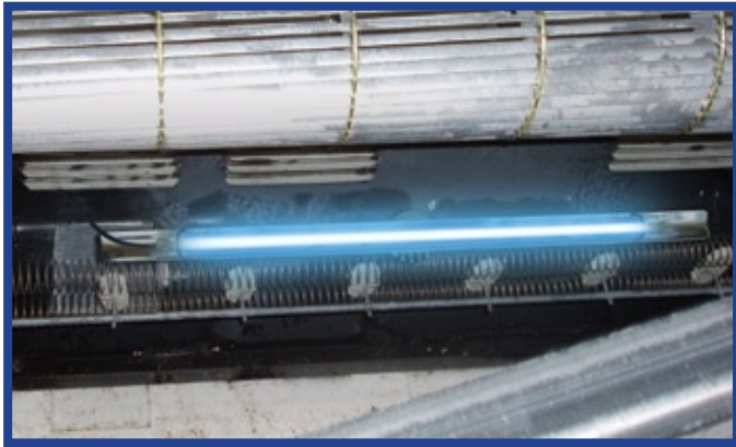
TIGHT FIT KIT UV™ installed in PTAC unit
