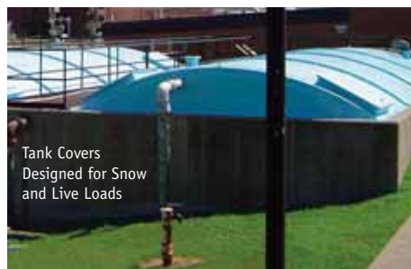
Underground Storage Tank
