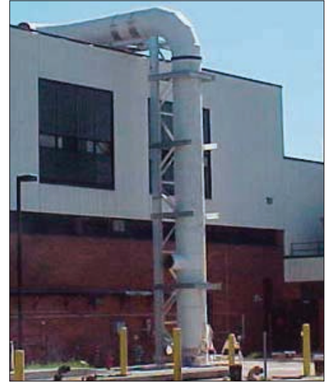
Odor control duct systems for water treatment
