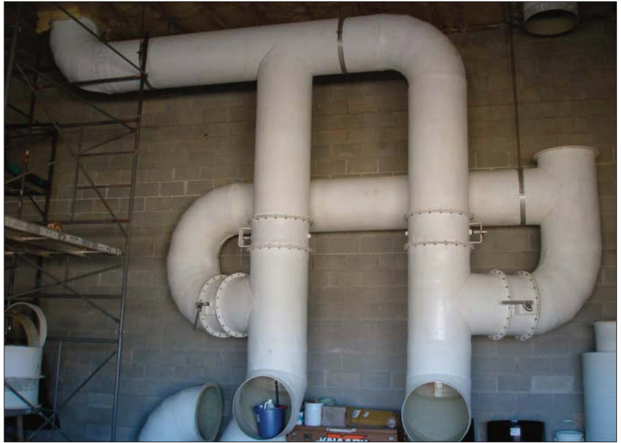
Prefabricated corrosion resistant duct system for water plant chlorine room
