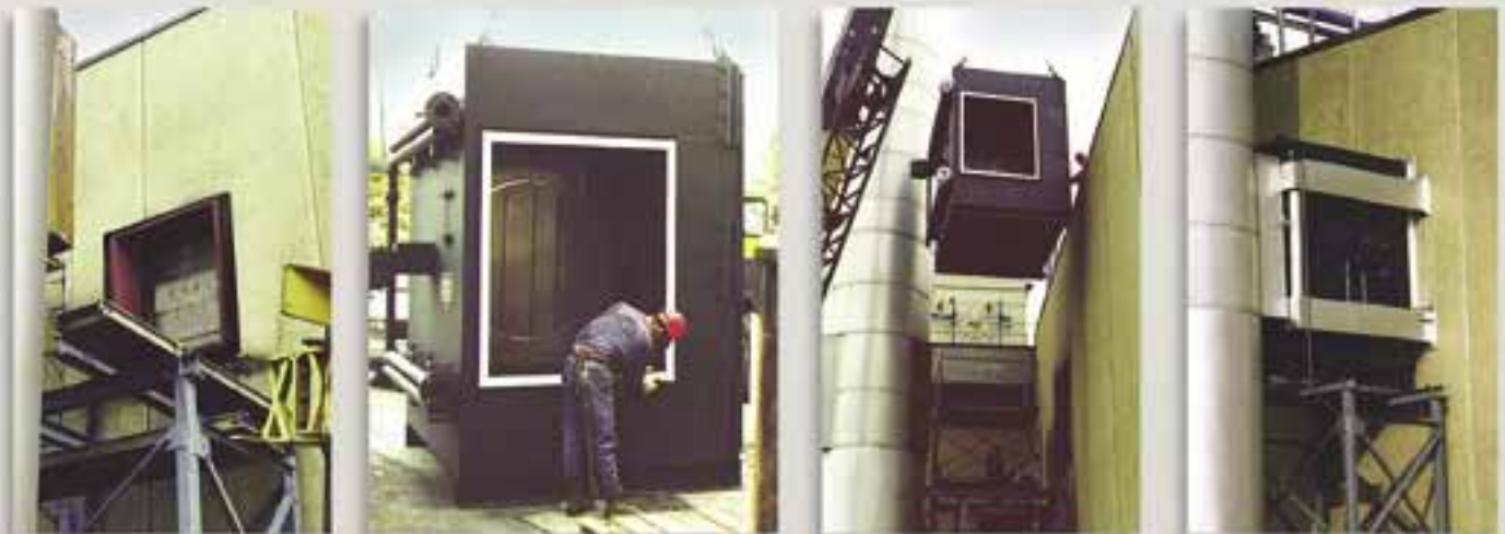
BREWERY, Ontario, Canada (1) RTR-1V2Q28CSS recovering Btu from (1) 95,000 pph steam boiler; Reducing 505°F @ 24278 SCFM to 333°F; Raising 196 gpm boiler feedwater entering at 225°F to 278°F.
