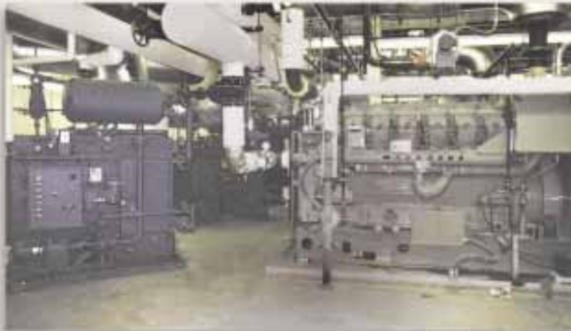
HOSPITAL , Chicago, Illinois (3) Model ESG1-616B18CSS. Recovering Btu from (3) Waukesha 3516, 1,100kW natural gas engines. Reducing each 2,392 SCFM from 1,135°F to 438°F. Delivering 2,173 pph steam @ 130 PSI operating (150 PSIG design).
