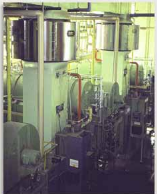
HOSPITAL , Flint, Michigan (2) FTR-160E28SSS each recovering Btu from (1) 435 BHP steam boiler; Reducing 450°F @ 4251 SCFM to 279°F; Raising 30 gpm boiler makeup water entering at 50°F to 109°F.
