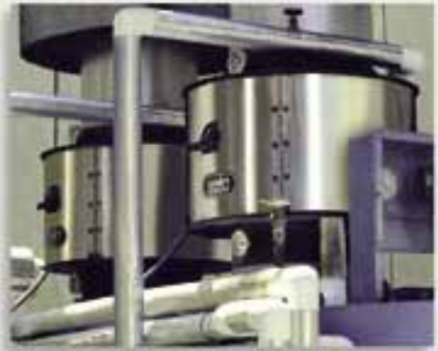
Condominium Complex, Milwaukee, Wisconsin EM Series economizer, on top a domestic hot-water heater, preheating municipal water.
