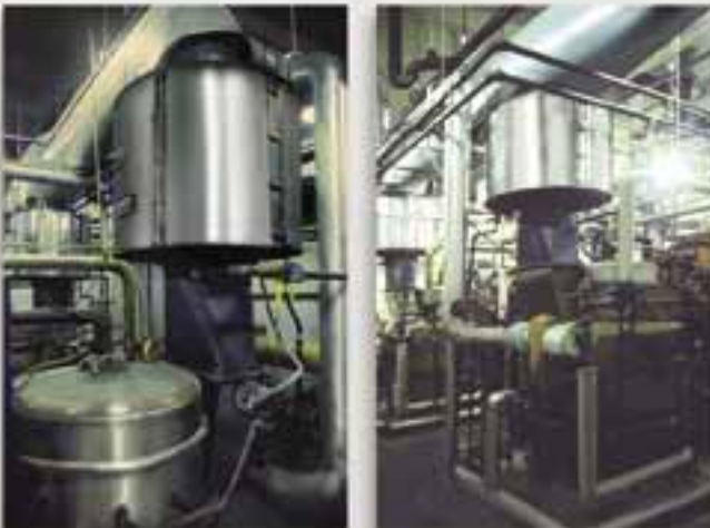
WASTE WATER TREATMENT PLANT, Fond du Lac, Wisconsin (2) FCR-1J2D25ALS each recovering Btu from (2) 150 BHP steam boilers; Reducing 700°F @ 1603 SCFM to 246°F; Raising 18 gpm boiler feedwater entering at 100°F to 201°F.
