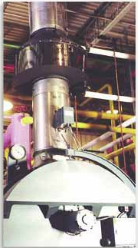
PRINTING FACILITY , Lomira, Wisconsin (2) Model: FCR-1L2C16ALS each Recovering Btu from a 500 BHP steam boiler; Reducing 400°F @ 4205 SCFM to 252; Raising 34.5 gpm boiler feedwater entering at 120°F to 164°F.
