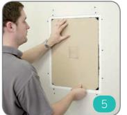
Secure product to installation block with one dry wall screw through the mounting hole at each corner of the product. Adjust screws to ensure front surface of loudspeaker is 1mm to 2mm behind the dry wall surface.
