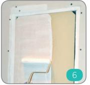
Apply a coat of PVA adhesive to the surface of the panel loudspeaker and to the area of dry wall stripped back around the product's perimeter. Allow to dry opening, filling the perimeter gap for a few minutes.
