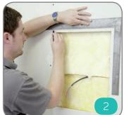
For optimal visual results, mark a Remove the paper around the studs the same size as the product second perimeter line approx. 3/4 perimeter of the aperture, and inch outside the perimeter of the chamfer with sanding block or series of shallow cuts. Add sound product aperture and score at an scraper to recess 1mm below inward angle just through the dry surface, allowing for a completely wall paper surface, or skip to #4. flush installation.
