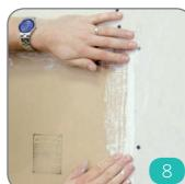
apply mesh or paper joint tape around the perimeter of the product, straddling the product and the stripped-back dry wall to create a filled, level backing for making sure not to overlap the paper edge of the drywall.
