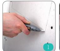
Create wall opening between by using a utility knife, making a insulation into cavity. Ensure cables are pulled into position.
