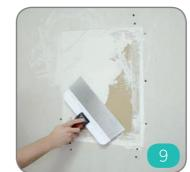
Apply skim-coats of dry wall compound across entire panel surface and the area of stripped back dry wall and at least 6 beyond the seam to minimal 3/16th (2mm) thick. (this might take 2 or 3 applications, let dry in-between).
