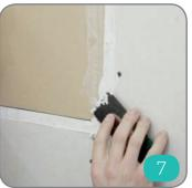
Using a taping knife or decorator While the compound is still wet blade, push dry wall compound down between the edge of the panel frame and the drywall the tape to adhere to.
