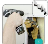
corner using two drywall screws secured through the front of the plasterboard in to the plastic lug provided. Connect loudspeaker cable and test operation.
