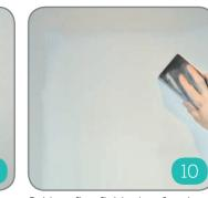
Achieve fine finished surface by sanding back/filling any lower spots and feathering the edges to create an undetectable transition. Paint or wallpaper surface with decoration of choice.
