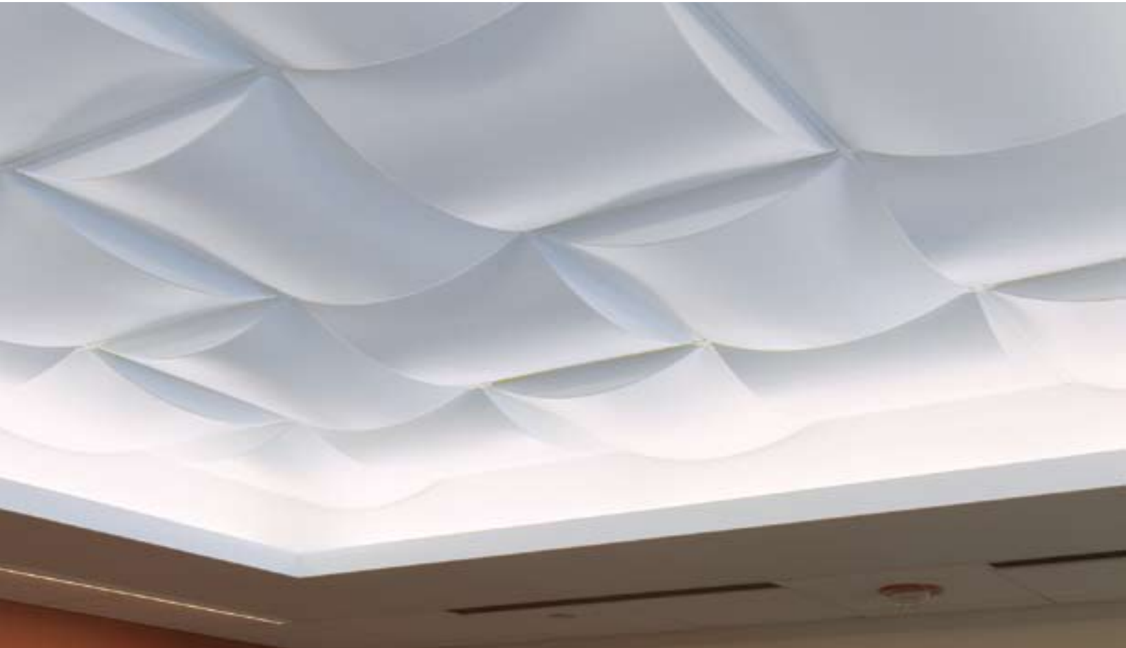
BILLO 3-Dimensional Panels, White Translucent and White Opaque/ DONN CENTRICITEE DXT Suspension System, Flat White
