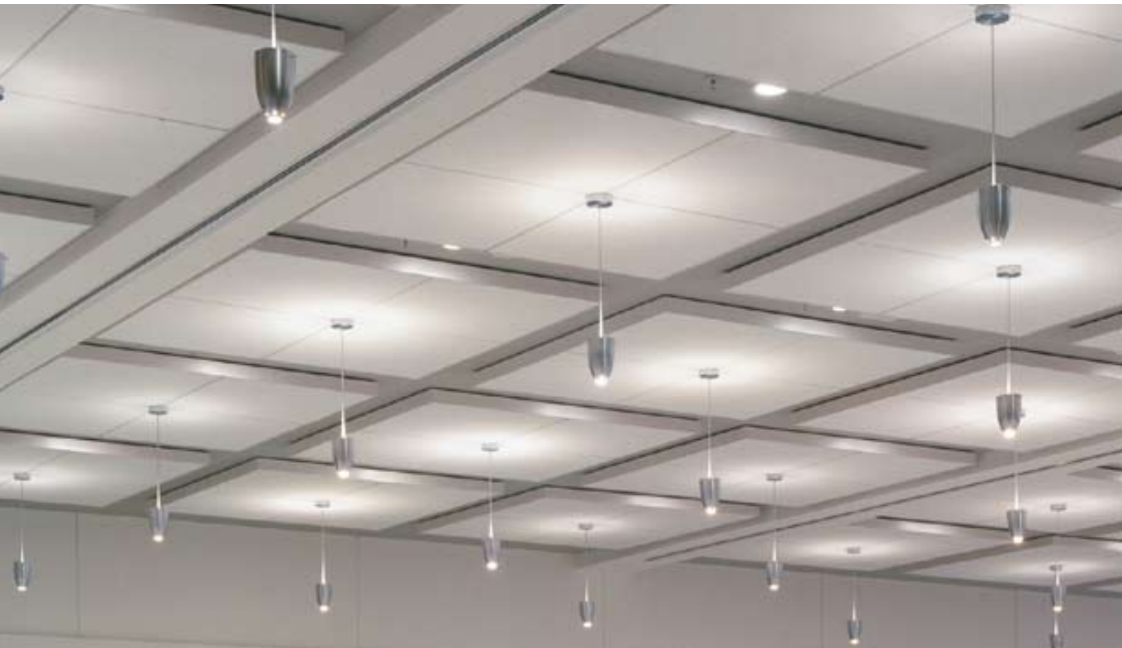
COMPASSO Perimeter Trim with HALCYON CLIMAPLUS Ceiling Panels/ DONN FINELINE DXF Suspension System
