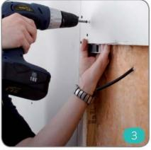
Fix installation lugs using two drywall screws secured through the front of the plasterboard into the plastic lug.
