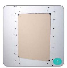
Position product in aperture. Connect loudspeaker to cable and test its operation.
