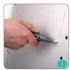
Create aperture using a sharp knife, making a series of shallow cuts. Add sound insulation into cavity.
