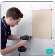
Secure product in place with one drywall screw through each corner of product. Adjust screws to ensure panel is flush with wall.
