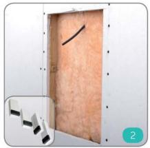
Position installation lugs under top and bottom corners of surrounding plasterboard. Ensure cables are pulled to this position.
