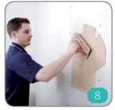
Skim with plaster (ordinary multifinish is fine). The best finish is produced when the entire wall is skimmed at the same time.
