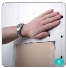
Apply joint tape, covering join between panel and plasterboard. Perform final electrical/audio test.
