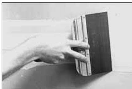
2. First Finishing Coat
