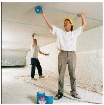
ProForm® BRAND Paper Joint Tape — Joint tape conceals and reinforces wallboard joints. The tape is buffed on both sides to ensure the best working qualities and bond. A center creasing process allows easy folding for use at corners. 75', 250' and 500' rolls.
