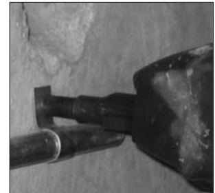
12HSMP034 clip assembly used to secure conduit
