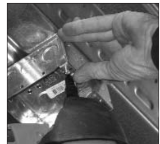
MP034TH fastener used to attach a junction box
