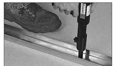
Track to floor
