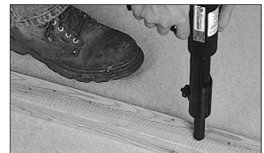
2" x 4" to concrete slab
