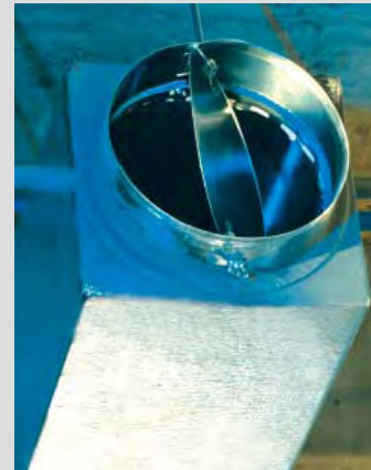
Below: Detail of installed duct with a fan at the end.
