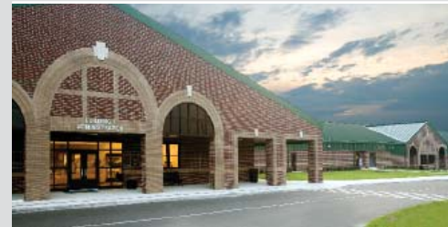
Oakleaf School in Clay County
