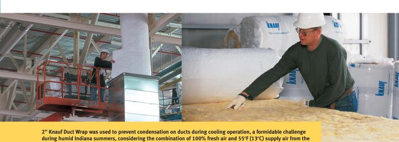
chillers. KwikStretch markings on the duct wrap helped installers make faster measurements.
