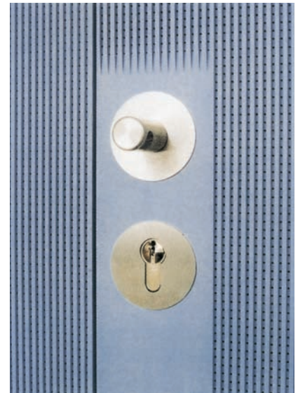
Painted Quadrillo cabinet doors with integral offsets for latch and locks.
