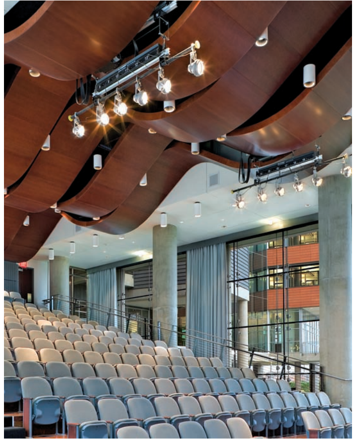
Quadrillo, custom toned ash panels in a direct suspended absorptive/reflective application met the stringent acoustical requirements of this auditorium.
