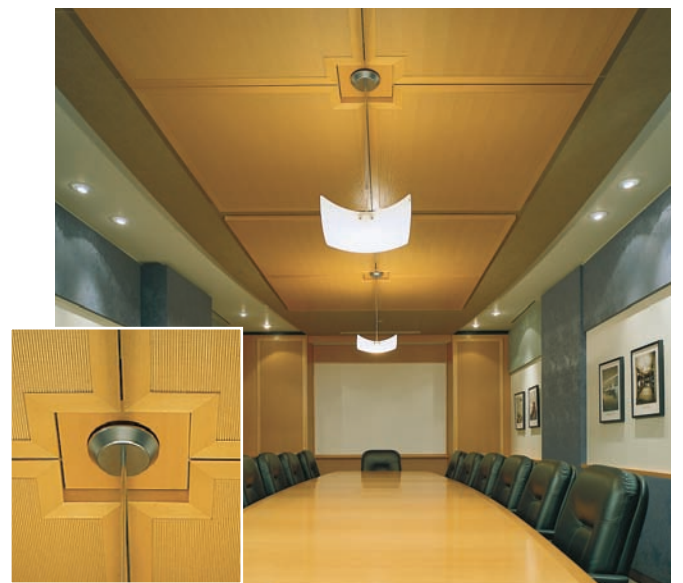
Custom Quadrillo ceiling with framed panels and a unique detail at light fixture suspension.
