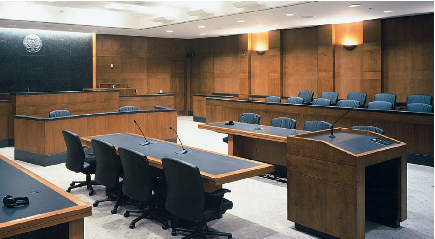
Quadrillo finished panels in five separate sections installed between pilasters on side walls.
