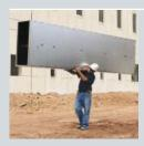
The Knauf KoolDuct System has only 15% of the weight of insulated sheet metal ductwork, so transporting and installing is easy and fast.
