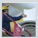
KwikFlex has excellent thermal properties, with low thermal conductivity ratings to 850°F (454°C).
