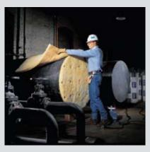
• Ideal for flat or irregular surfaces, especially for applications requiring a more flexible insulation.
