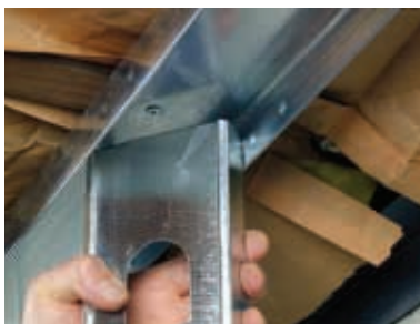
INSERT STUD IN WAREWALL® TRACKS & TWIST IN PLACE...NO SCREWS REQUIRED
