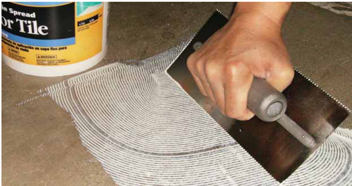
S-515 moisture-resistant adhesive being spread with recommended fine-notch trowel.
