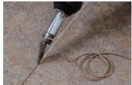
Weld rod seam
