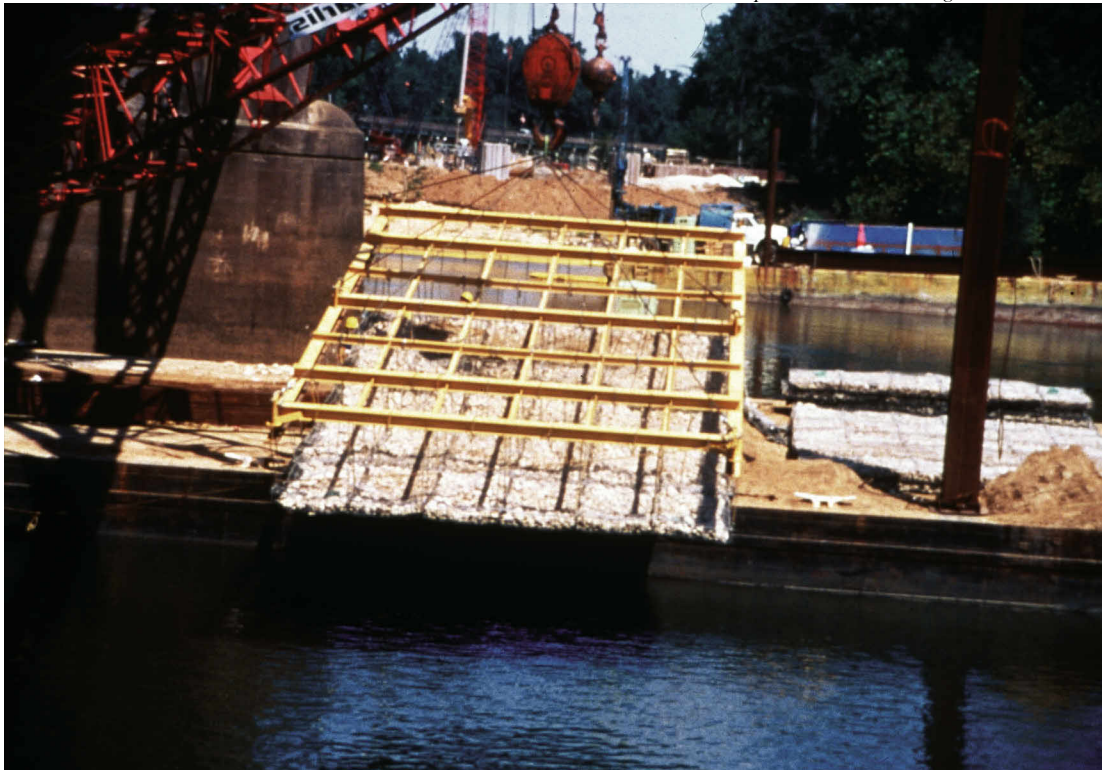
Apalachicola River Bridge, FL, Florida DOT
