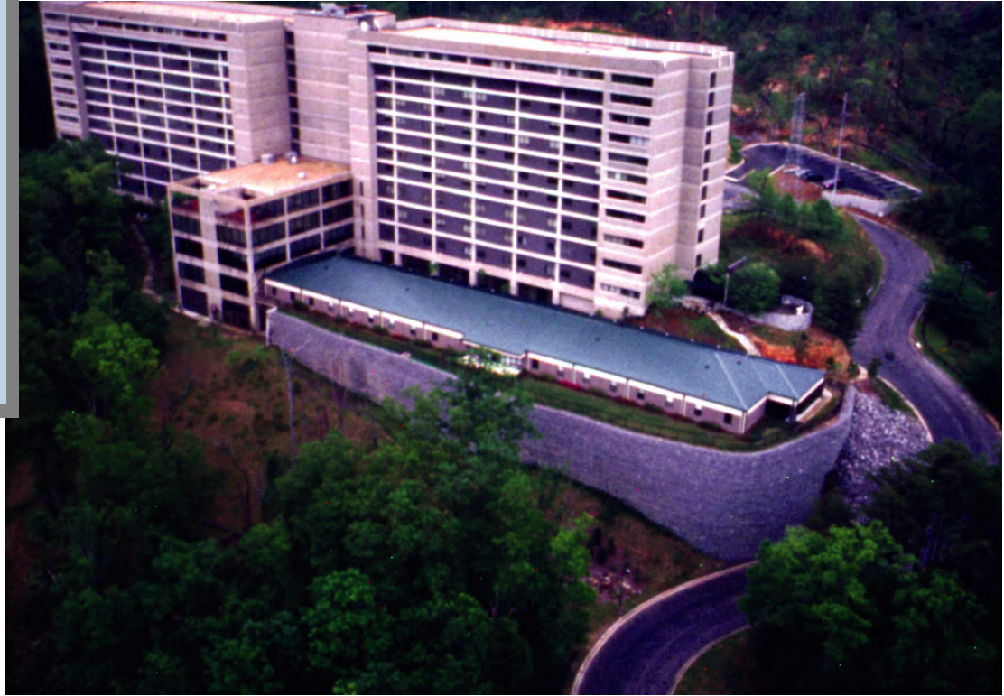
MSE Wall in Vestavia Hills, AL - Private property owner
