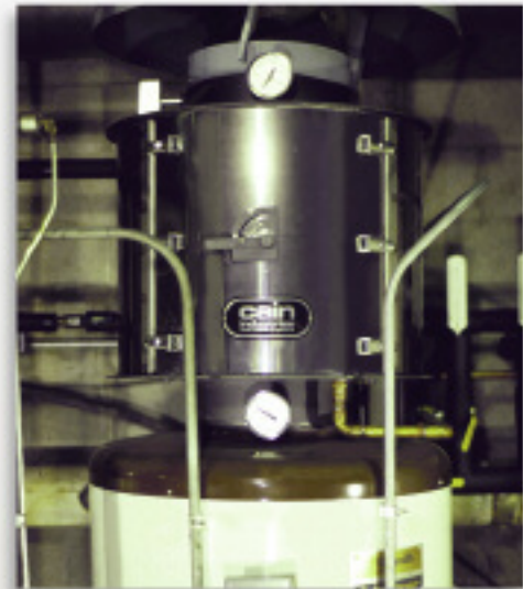
Condominium Complex, Milwaukee, Wisconsin EM Series economizer, on top a domestic hot-water heater, preheating municipal water.
