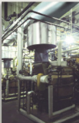
WASTE WATER TREATMENT PLANT, Fond du Lac, Wisconsin (2) FCR-1J2D25ALS each recovering Btu from (2) 150 BHP steam boilers; Reducing 700°F @ 1603 SCFM to 246°F; Raising 18 gpm boiler feedwater entering at 100°F to 201°F.
