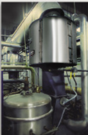
WASTE WATER TREATMENT PLANT, Fond du Lac, Wisconsin (2) FCR-1J2D25ALS each recovering Btu from (2) 150 BHP steam boilers; Reducing 700°F @ 1603 SCFM to 246°F; Raising 18 gpm boiler feedwater entering at 100°F to 201°F.
