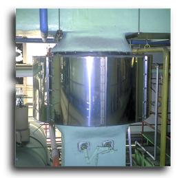
Stainless Steel Hinged Door – Panels For Immediate Access (requiring no tools)
